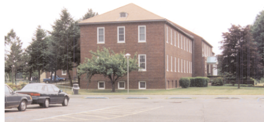
Figure 142. View of Caumsett from parking lot
