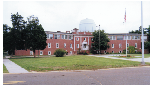
Figure 38. Kreiling with water tower in distance
