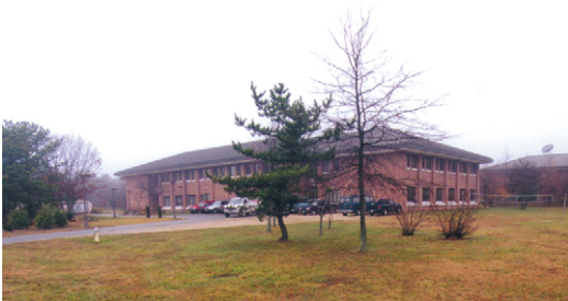
Figure 105. Service side of building
