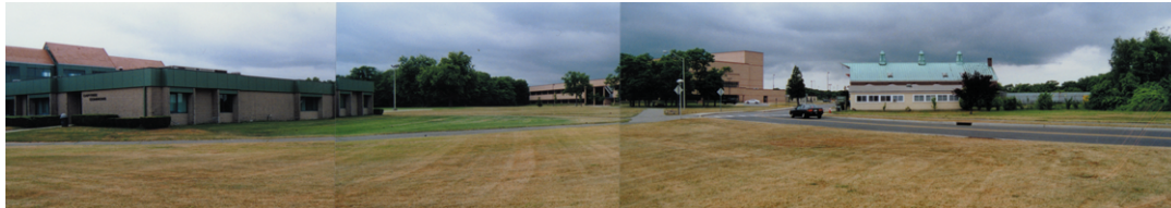
Figure 25. Panorama of Captree, Sagtikos and Plant Operations Buildings
