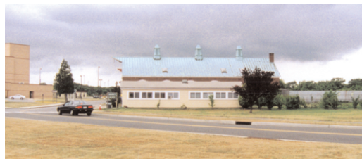
Figure 172. Plant operations building with storage building in foreground
