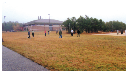
Figure 117. Central Energy Plant with volleyball courts in foreground
