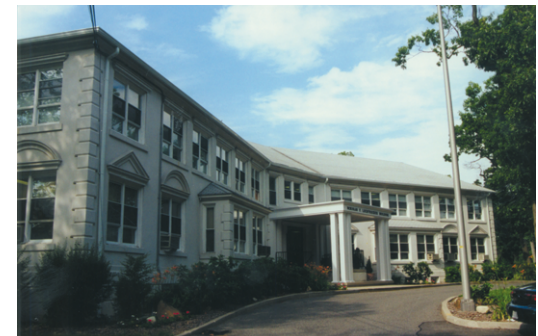
Figure 5. N.F.L. Central Administration Building.
