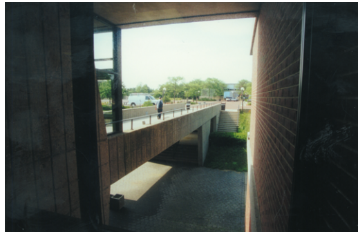
Figure 47. View of bridge from inside Riverhead
