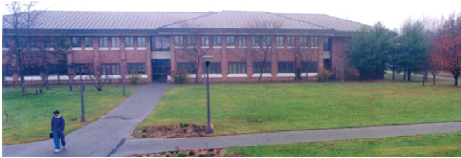
Figure 96. Quadrangle side of building
