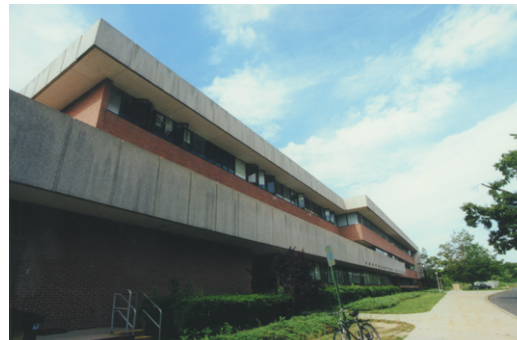
Figure 68. South side of Southampton and entrance at first flr
