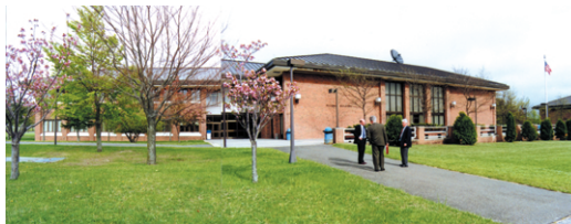
Figure 88. Facade facing quadrangle
