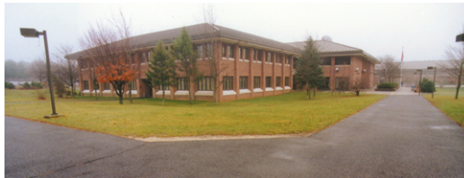
Figure 89. Peconic from north
