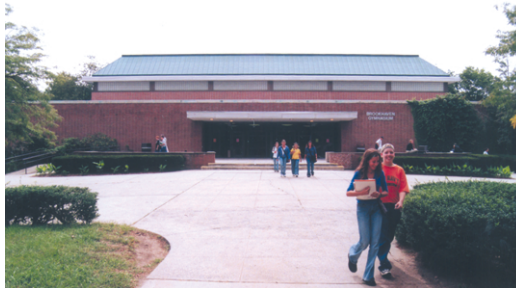
Figure 20. Main entrance at second floor
