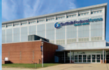
Suffolk Federal Credit Union Arena Michael J. Grant Campus, Brentwood, NY
